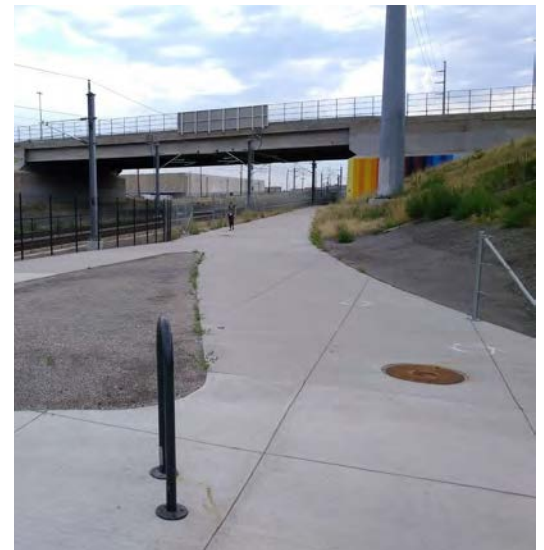
A shared use path leads directly from the 40th and Colorado Station to a large multi-family residential development, but there is no wayfinding signage to communicate this.
